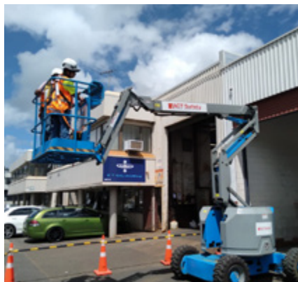
Elevated Work Platform Training
